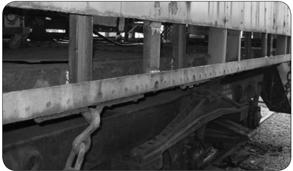
*New side supports have been welded into place to support both the exterior side sheets and the interior walls. Jan. 27, 2006. (Photo by Michael Steinberg.)*
